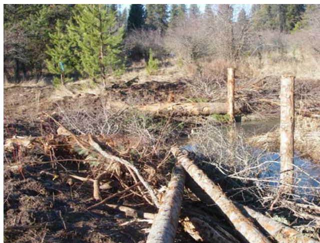
Same bank after restoration
