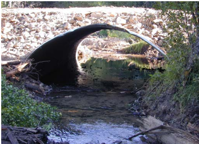
Stream crossing after culvert was installed
