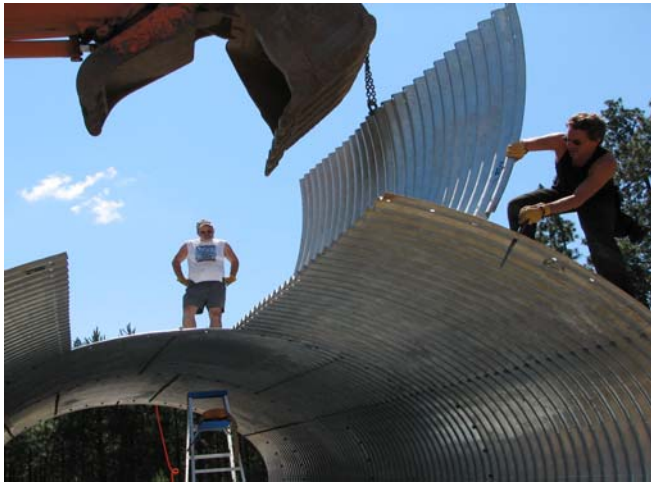
Jeff Jordan & Dan Jolibois install the last plate on culvert
