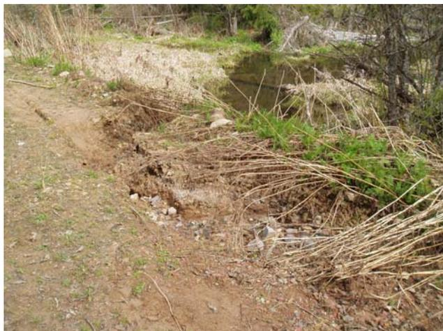
Figure 1. Example of an eroding roadbed where sediments are being delivered directly to the adjacent creek.
