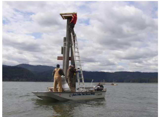
A new nesting platform is attached to a piling.
